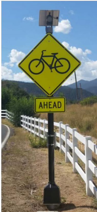
Example of dynamic warning system (Source: Dynamic Warning System to Alert Motorists to the Presence of Bicyclists )
