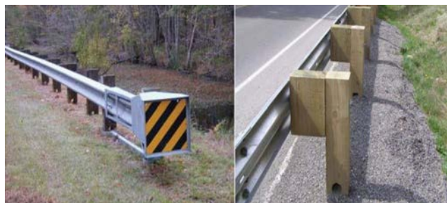
RD26: Example of guardrail application (Source: ODOT Crash Reduction Factor Manual)
