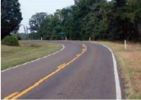
RD14: Example of post-mounted curve delineators (Source: ODOT Crash Reduction Factor Manual)
