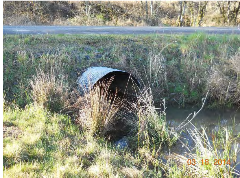
Photo 2: Inlet of Old Reservoir Road culvert
