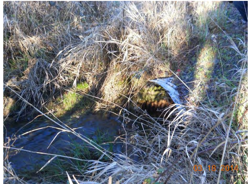
Photo 4: Outlet of Old Reservoir Road culvert
