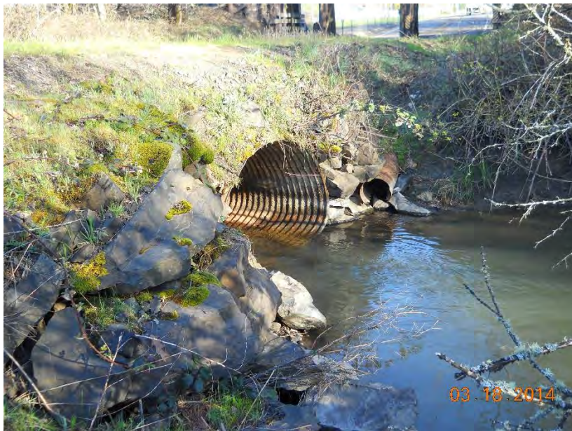
Photo 11: Outlet of 53 rd Street culvert
