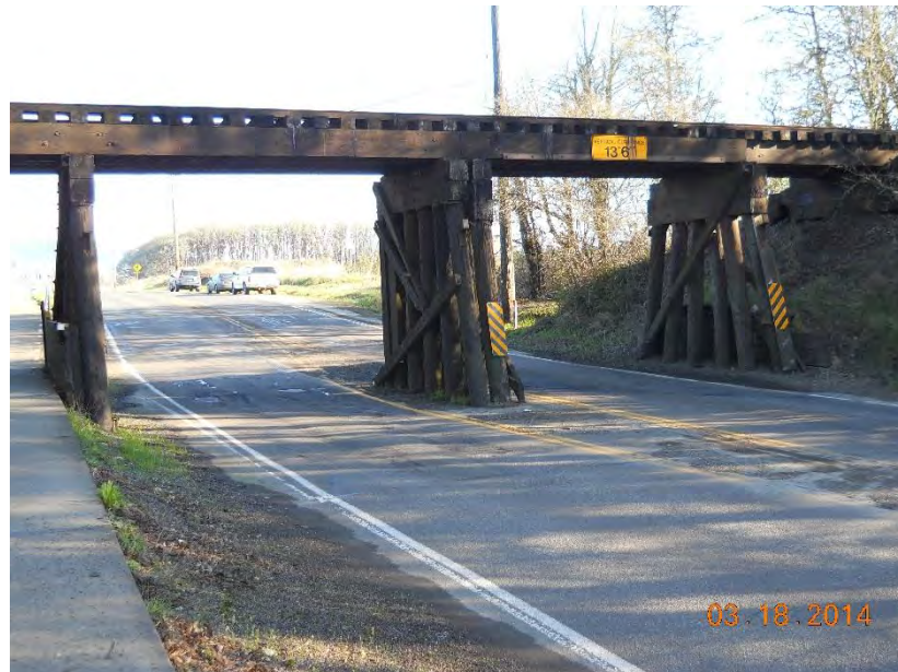
Photo 7: Railroad bridge over 53 rd Street
