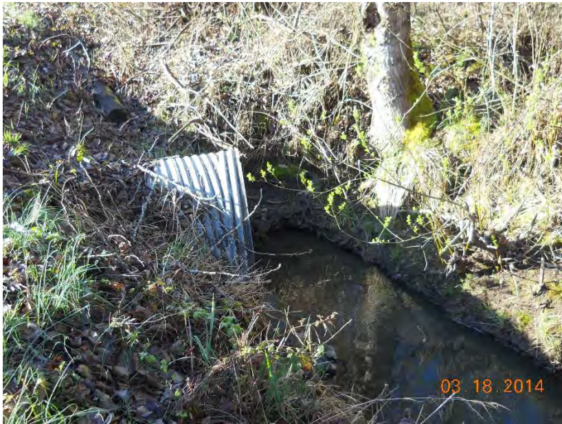
Photo 9: Inlet of 53 rd Street culvert
