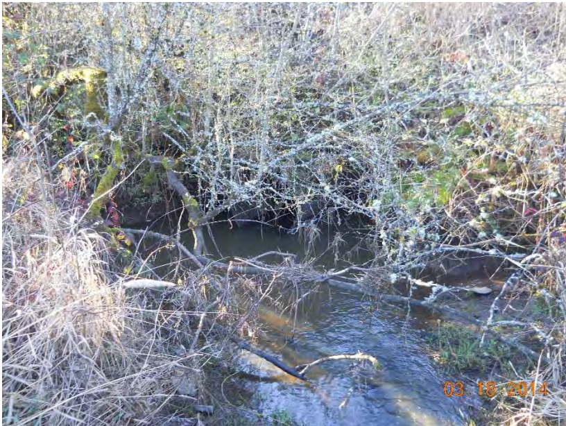
Photo 3: Inlet to railroad culvert
