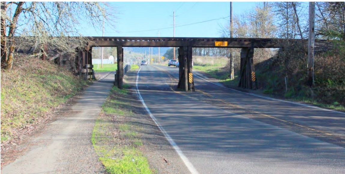
Figure 3. Existing Railroad Bridge, looking north
