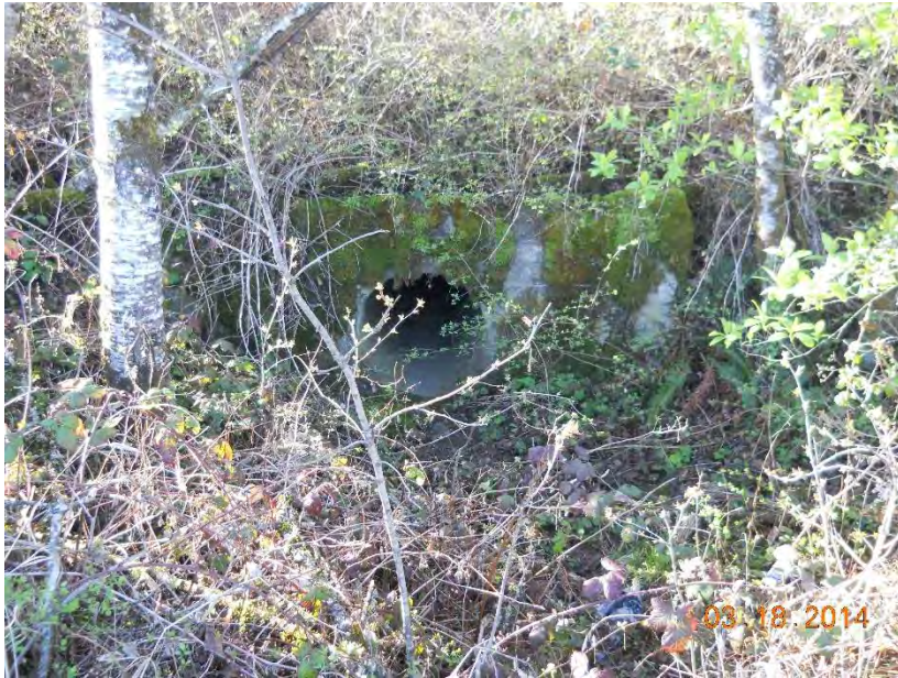
Photo 5: Inlet of railroad overflow culvert
