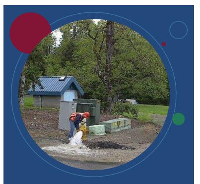
System Operators flush water lines and fire hydrants twice a year to help maintain water quality.
