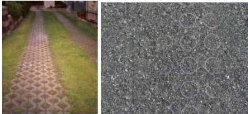
Residential driveway (Source: R. Bannerman); Plastic grid filled with gravel (Source: Gravelpave ® )
