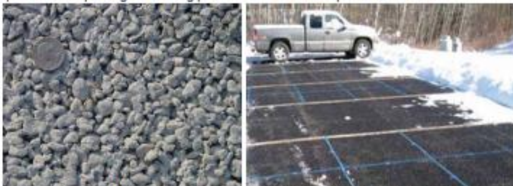
Pervious concrete (Source: Hunt and Collins, 2008); Porous asphalt parking lot (Source: University of New Hampshire Stormwater Center)
