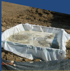
PLASTIC LINED WASHOUT
