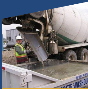
ROLL-OFF CONTAINER WASHOUT
