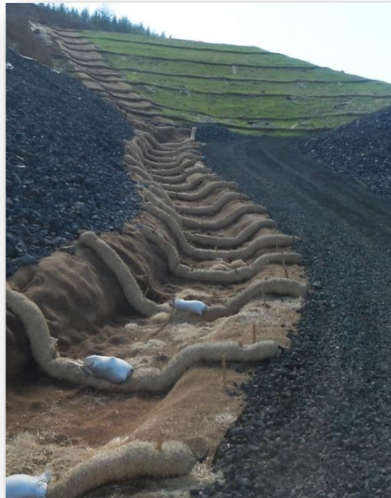
Figure 2-12 Stabilized Channel
