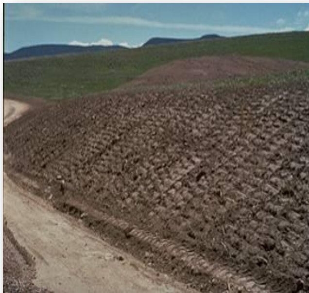
Figure 3-3 Roughened Soil Surface
