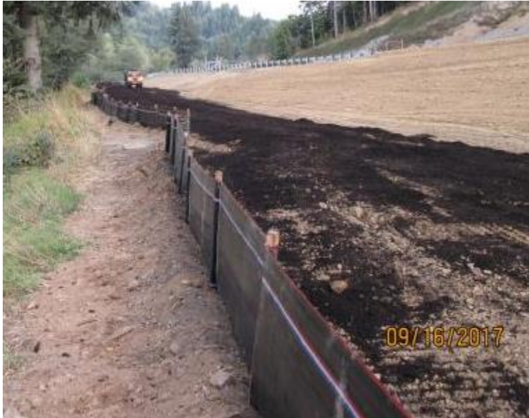
Figure 3-27 Sediment fence is trenched in correctly
