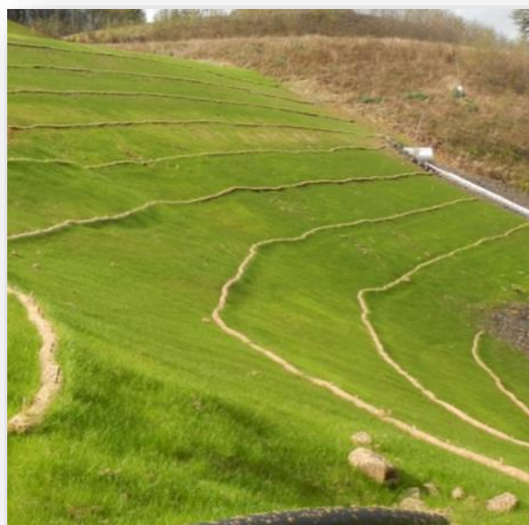
Figure 2-10 Seeded perennial rye grass with wattles to shorten slope length
