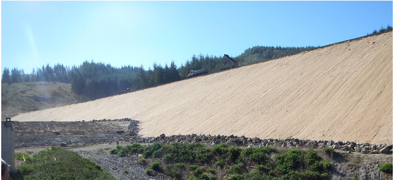
Figure 3-10 fully biodegradable slope protection matting
