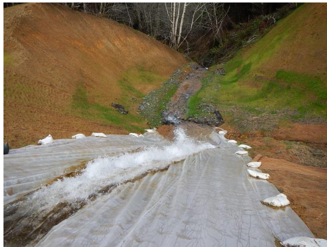
Figure 3-15 Plastic sheeting used as Temporary Slope Drains
