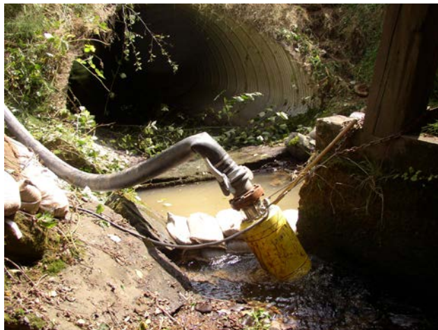
Photo examples of pumped bypass
