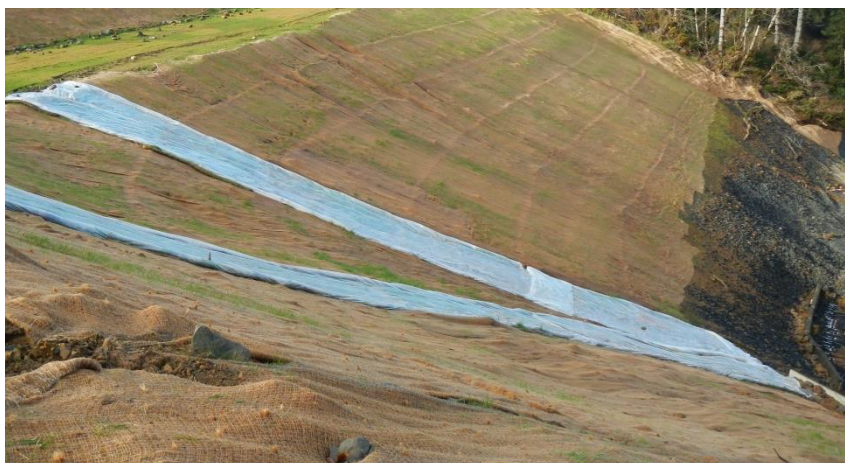
Figure 3-13 Plastic sheeting runoff control on slope matting
