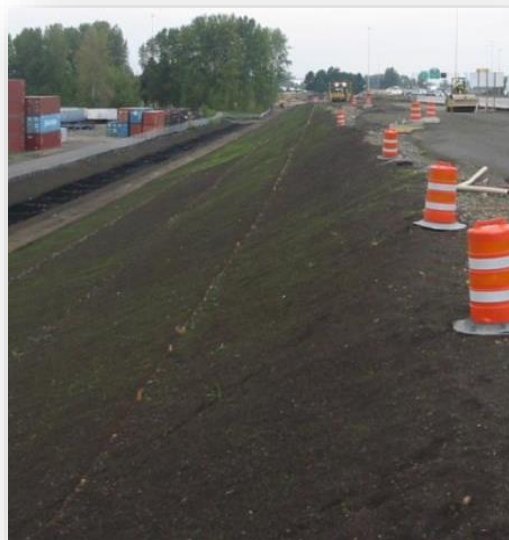
Figure 2-9 Compost blankets provides erosion prevention
