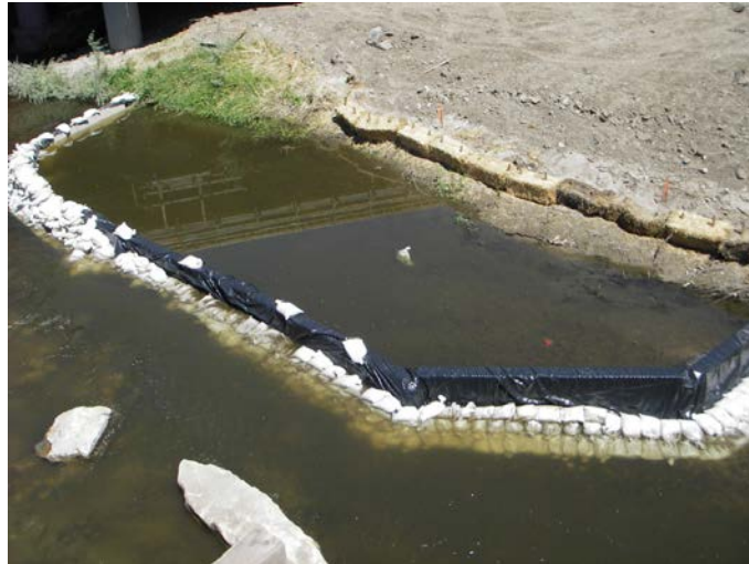
Photo example of Concrete Barriers with Sandbags
