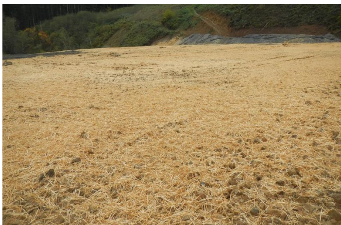
Figure 3-6 Good cover with straw mulch
