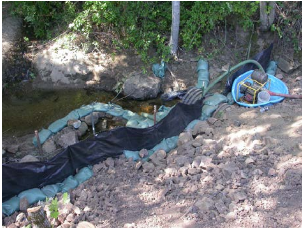
Photo examples of Temporary Water Management facilities
