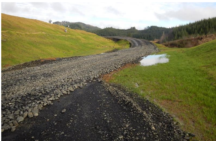
Figure 3-21 Stabilized Haul Road
