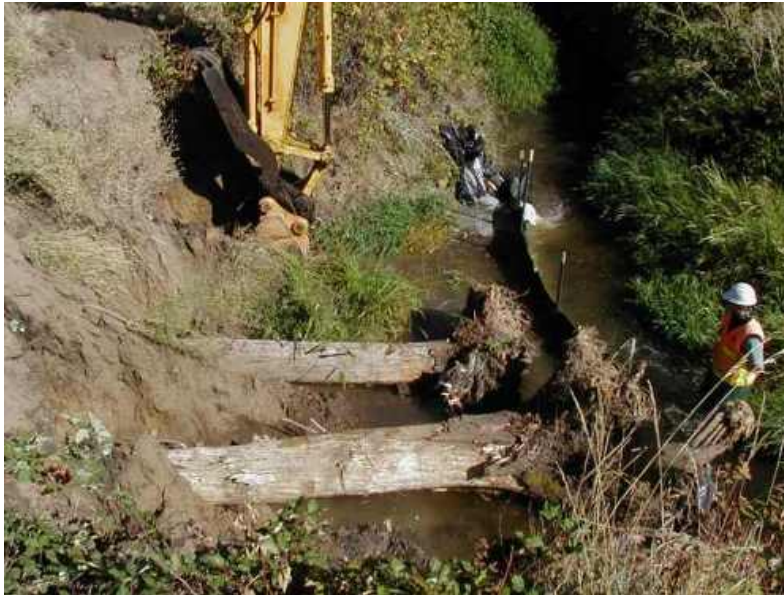
Photo example of Working in the Wet
