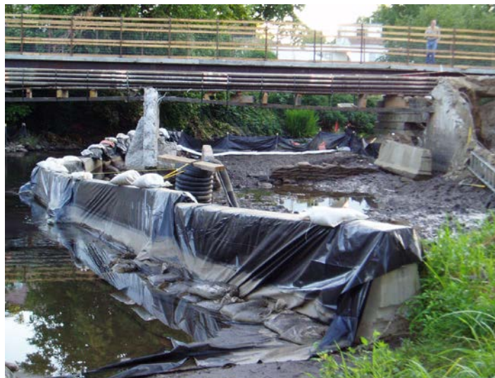
Photo example of Partial Isolation with Concrete Barriers
