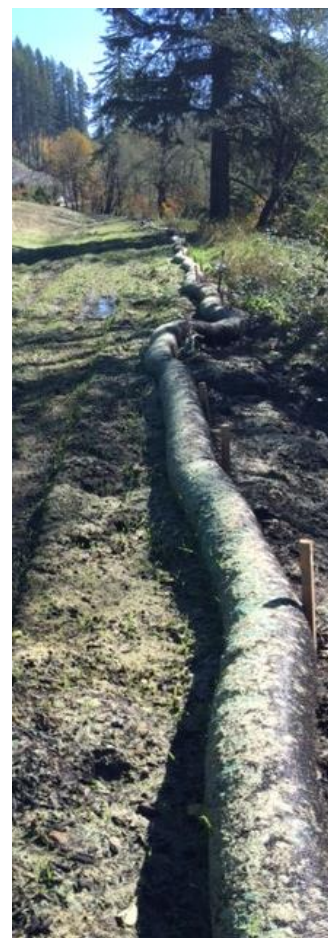
Figure 3-23 Compost Sock – Sediment Barrier Type 8
