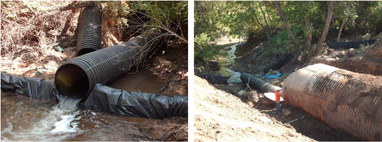
Photo examples of piping the stream flow through the existing structure
