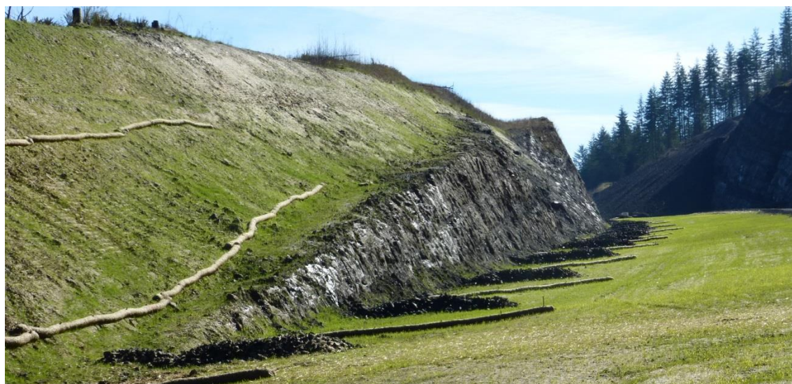
Figure 2-1 Good Sediment Control
