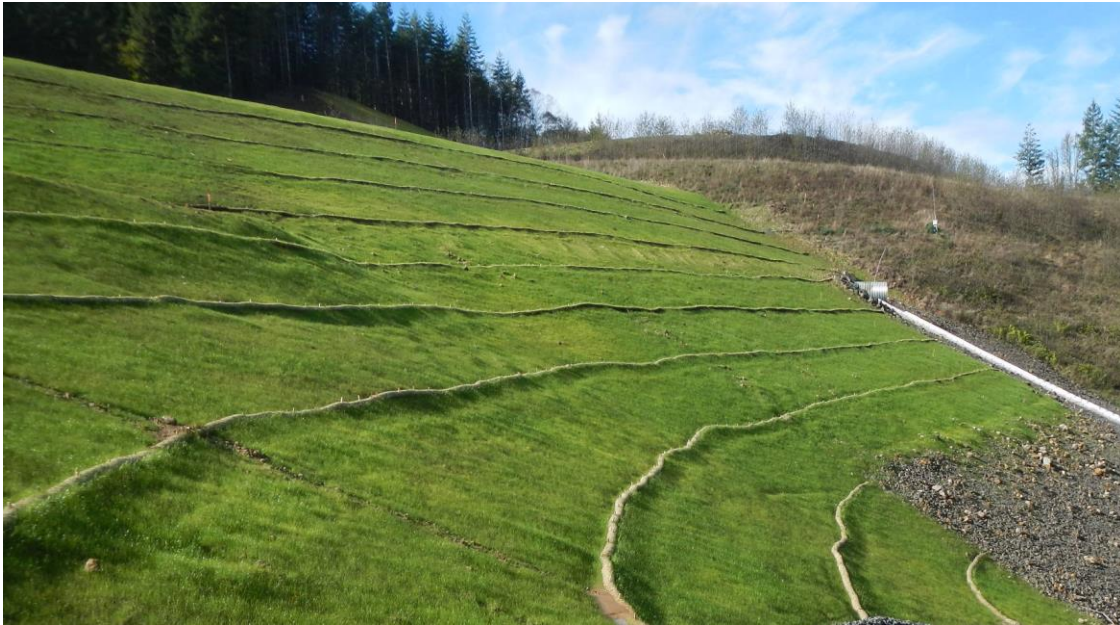
Figure 1-1 Fiber rolls shorten slope length and grass covers soil, preventing erosion
