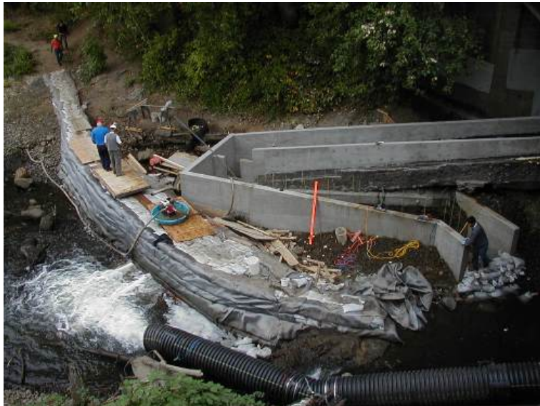
Photo example of Full Isolation
