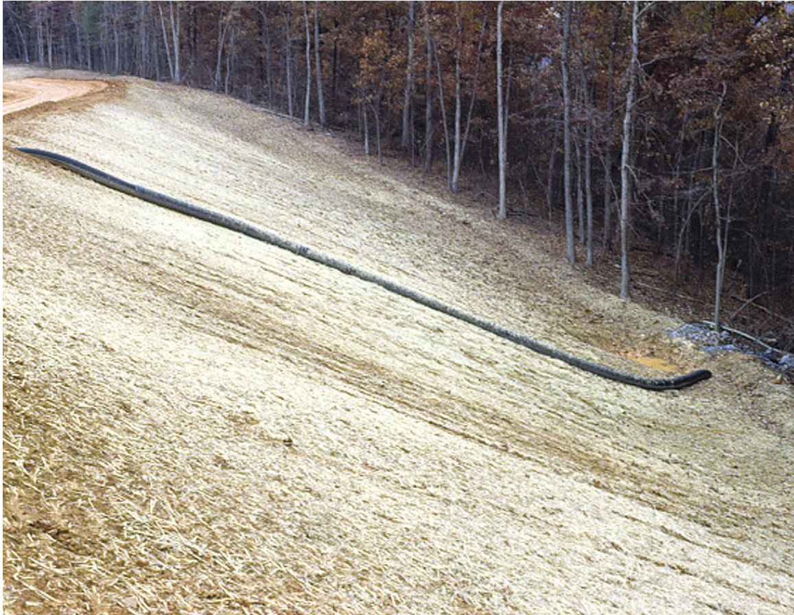
Figure 3-14 Temporary Slope Drains
