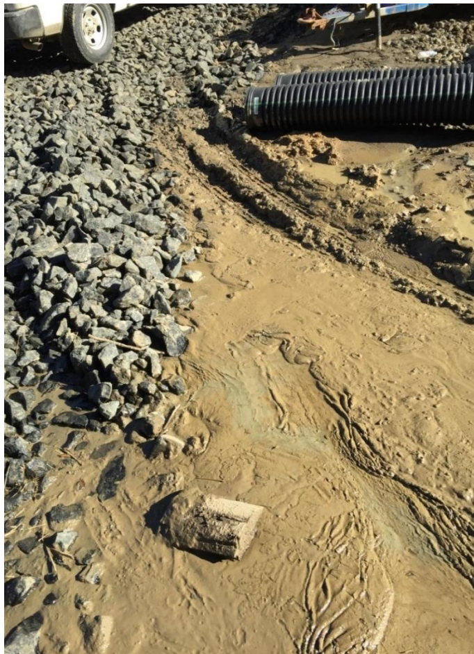
Figure 2-6 Sediment Non-Compliance
