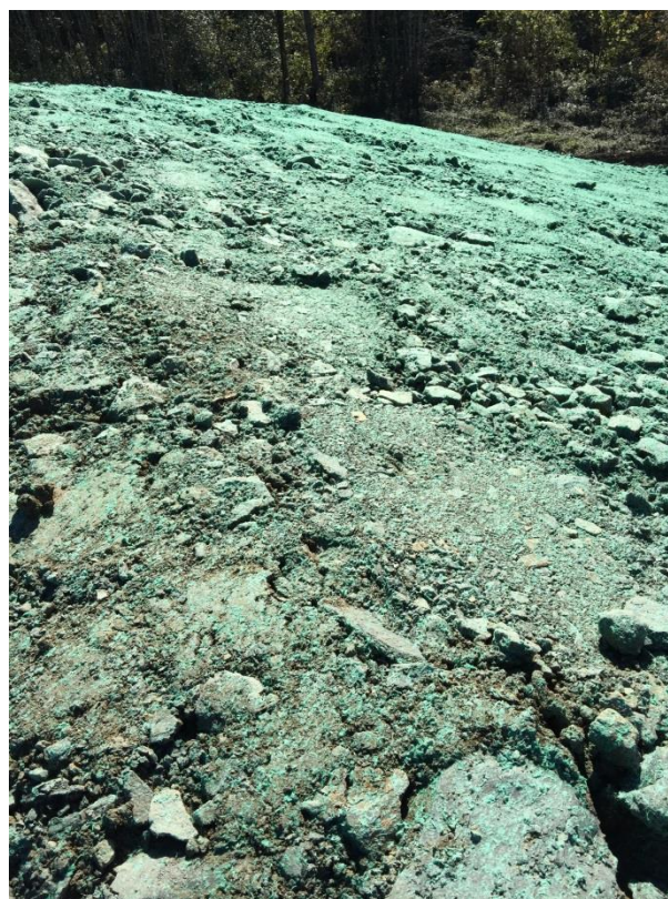
Figure 3-7 Thin hydromulch application
