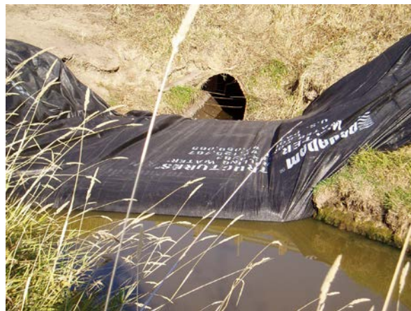
Photo example of Water Filled Impervious Membrane
