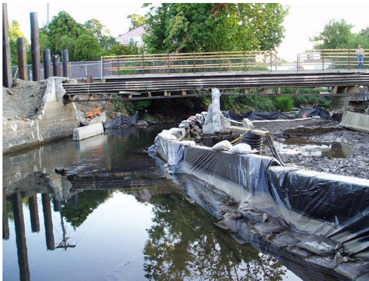
Photo example of Partial Isolation
