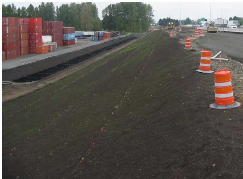
Figure 3-12 Compost blankets provides erosion prevention
