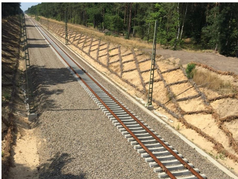
Figure 3-24 Novel brush barrier (brush wattles) Installation in Germany
