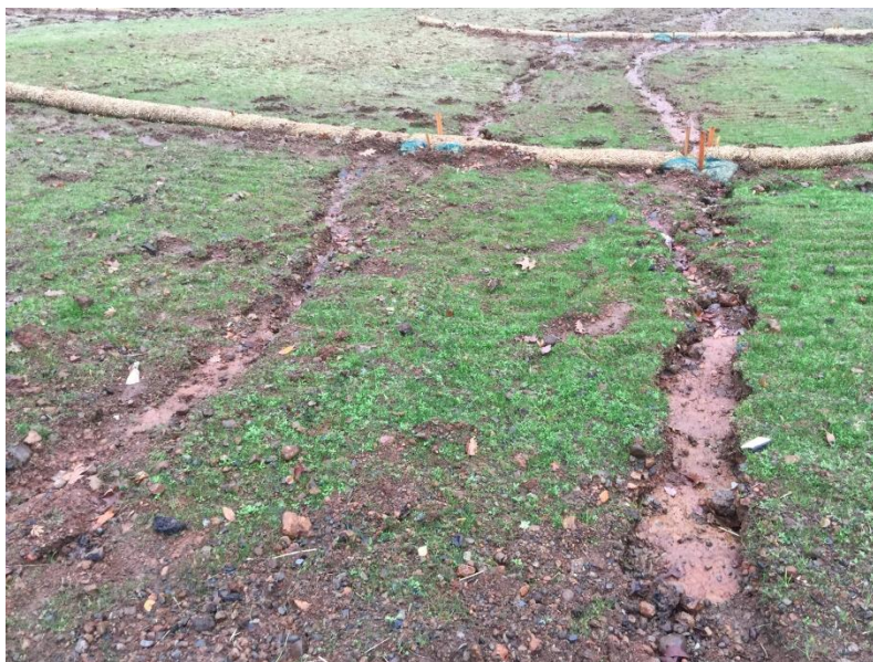
Figure 2-4 Rills on a Slope
