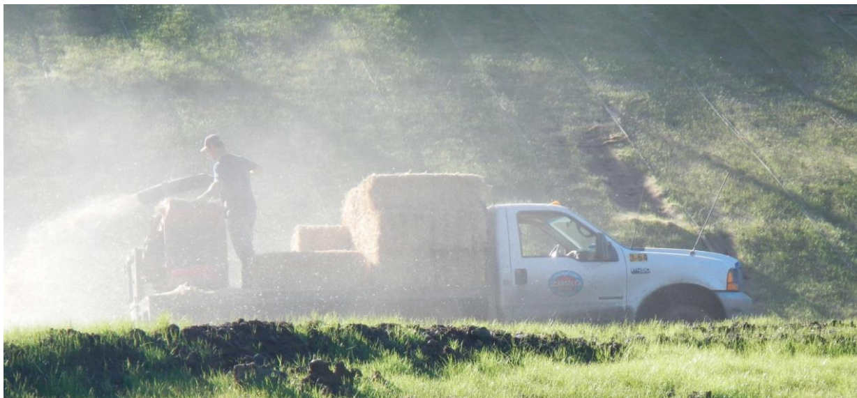
Figure 3-5 Straw Mulch being blown on site
