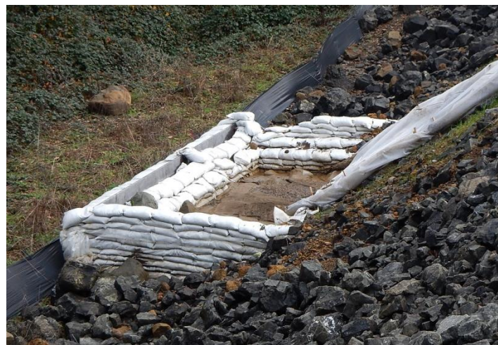
Figure 2-13 Sediment Trap & Energy Dissipater W/ Level Spreader
