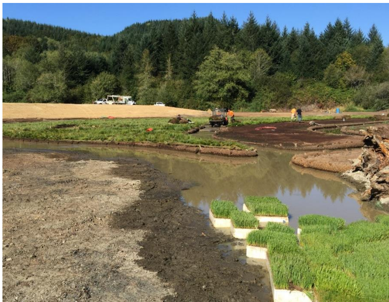
Figure 3-9 Installation of wetland sod
