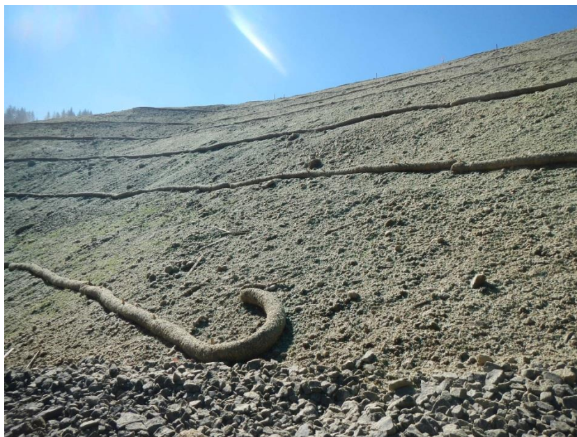
Figure 3-22 Fiber Rolls (Wattles) – Sediment Barrier Type 3
