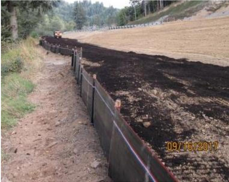
**Figure 3-27 Sediment fence is trenched in correctly**
