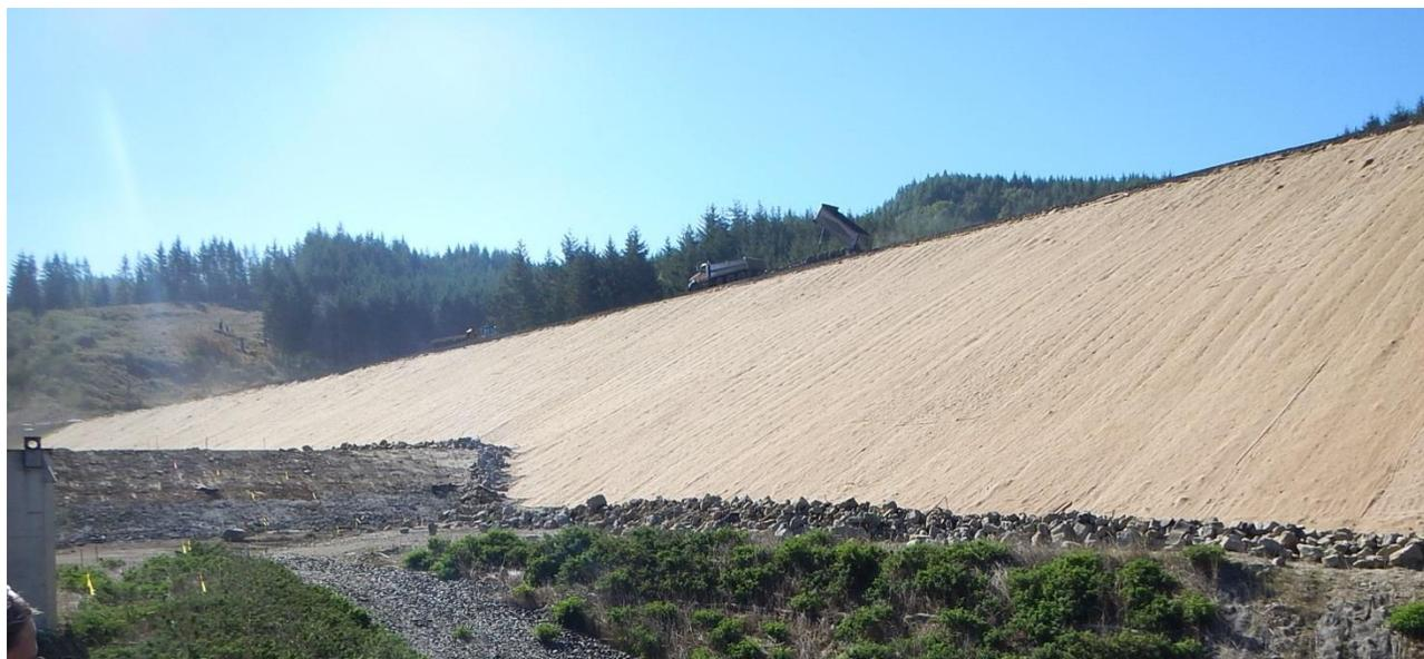
Figure 3-10 fully biodegradable slope protection matting
