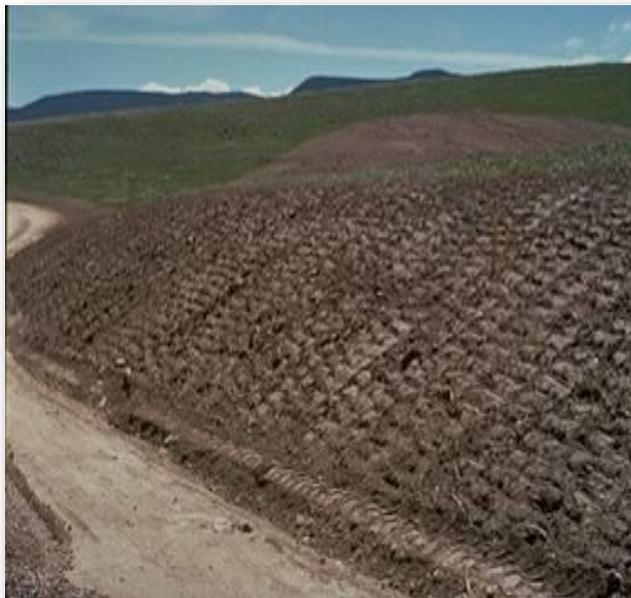
**Figure 3-3 Roughened Soil Surface**
