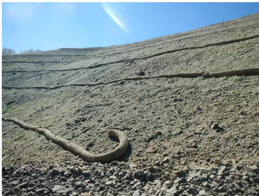
**Figure 3-22 Fiber Rolls (Wattles) – Sediment Barrier Type 3**
