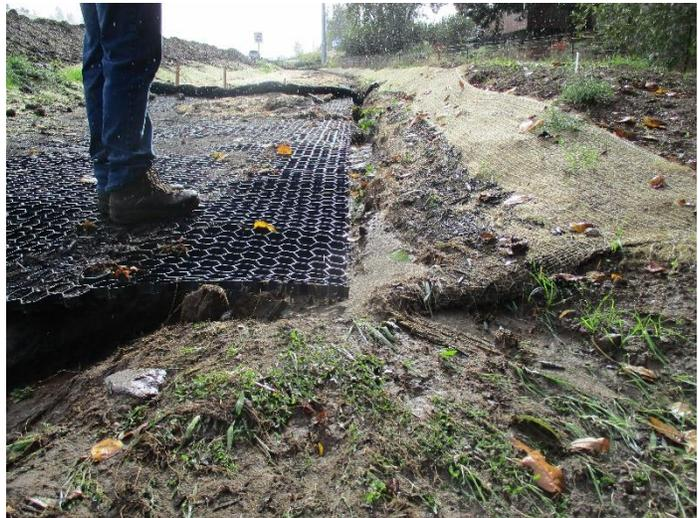
**Figure 2-7 Erosion control failure at water quality facility**
