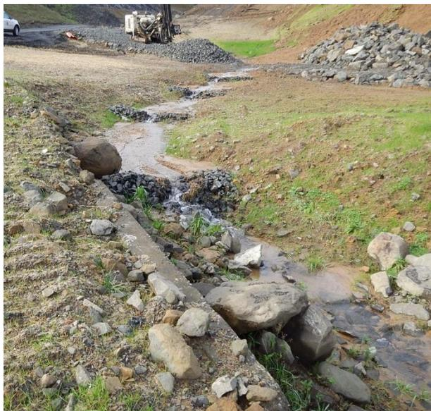
**Figure 2-11 Check Dams slow runoff velocity**
