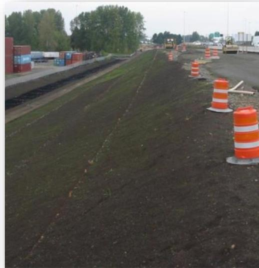
**Figure 2-9 Compost blankets provides erosion prevention**
