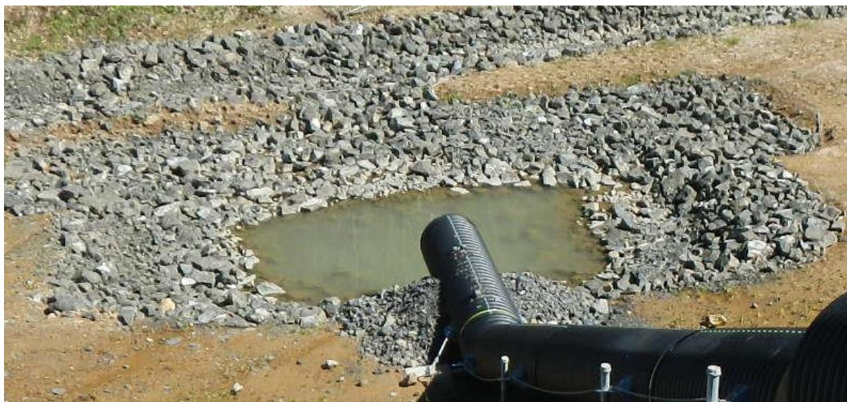
Figure 3-16 Energy Dissipater (permanent installation)
