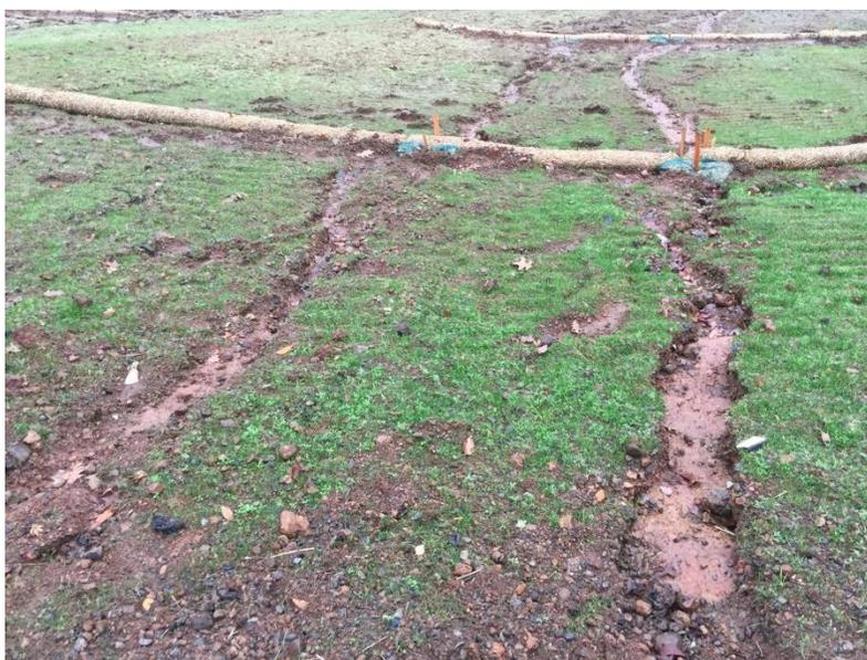
Figure 2-4 Rills on a Slope
