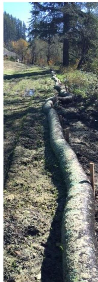
**Figure 3-23 Compost Sock – Sediment Barrier Type 8**
