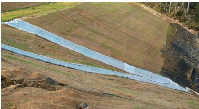
**Figure 3-13 Plastic sheeting runoff control on slope matting**
