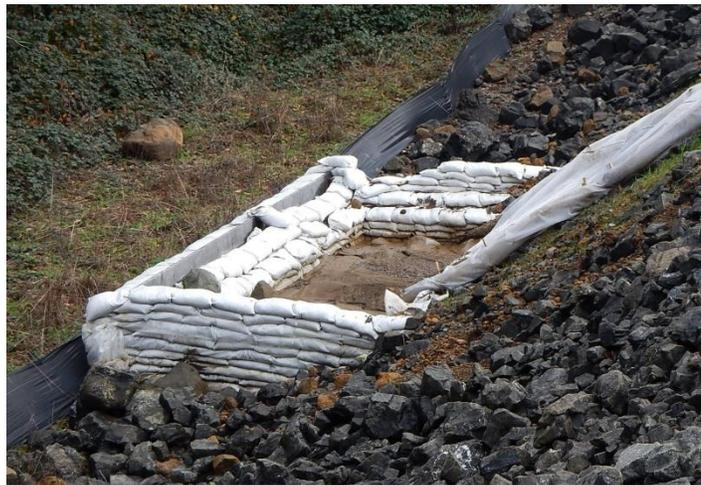
**Figure 2-13 Sediment Trap & Energy Dissipater W/ Level Spreader**
