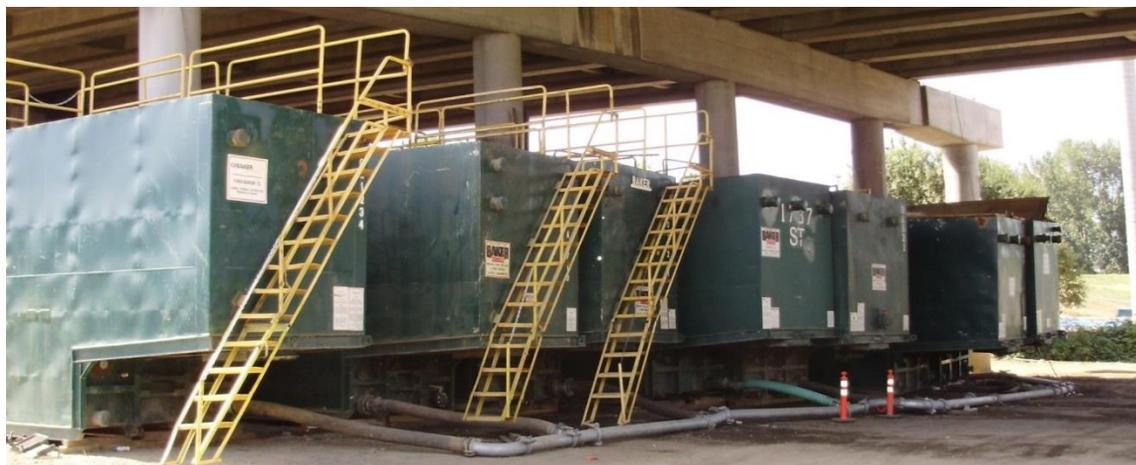
Array of Baker Tanks provide treatment to settle out the sediment, storage and filtration to ensure discharged water is clear.
