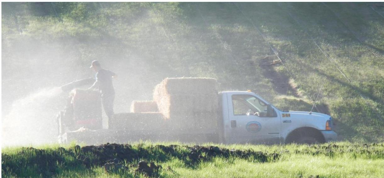
**Figure 3-5 Straw Mulch being blown on site**
