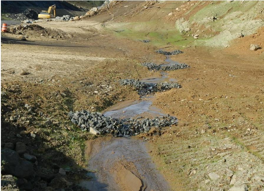
Effective functioning check dams with sediment impounded behind each dam.
