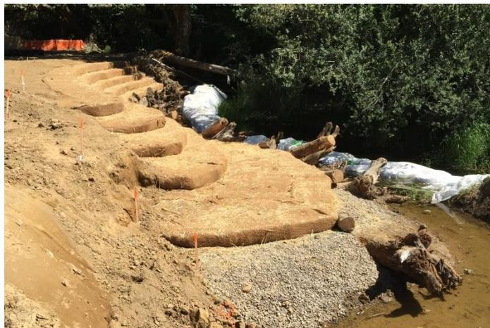
Woven coconut fiber matting (coir) with compacted coir "face" stabilizes stream bank soils. Embedded large wood deflects flows, slows velocity along shore margin and provides calmer micro-habitat for juvenile fish
