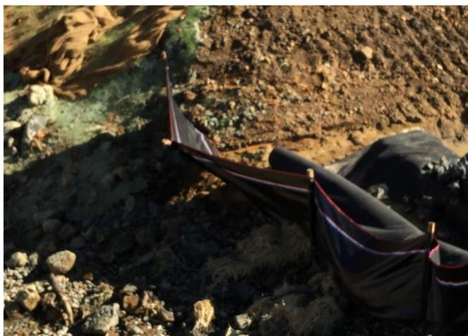
**Figure 3-30 Sediment fence not embedded in ground**
