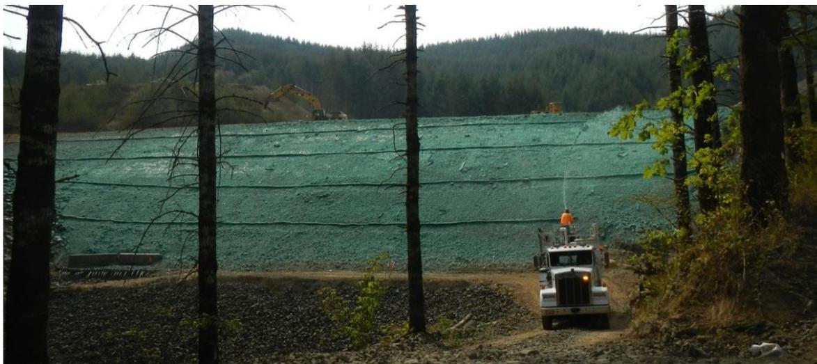
**Figure 3-4 Seeding & mulch applied with Hydroseeder**
