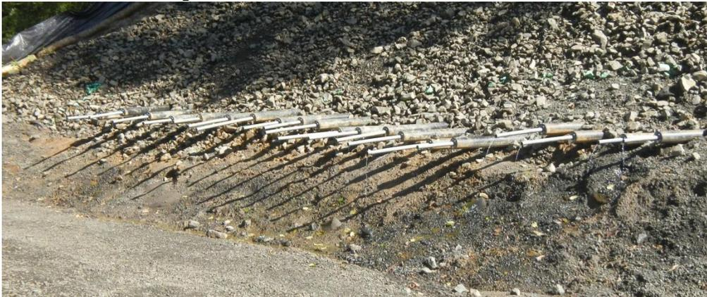
Water adds weight and lubrication to the structure of slopes that can result in landslides. Removing that water helps stabilize slopes especially in landslide prone locations. Horizontal drains (shown) can be drilled into hillsides. Drain boards can be layered into the construction of embankment slopes to help water exit those structures.
