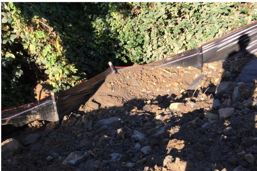
**Figure 3-29 Sediment fence maintenance failure**
