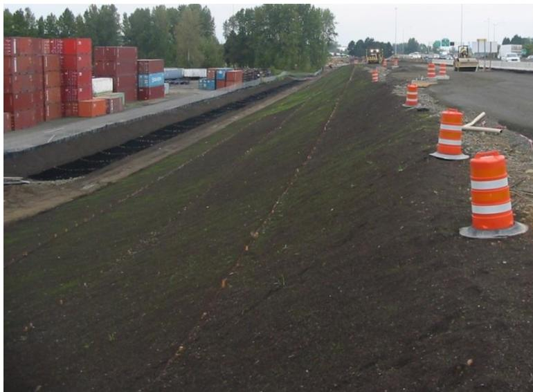
Figure 3-12 Compost blankets provides erosion prevention
