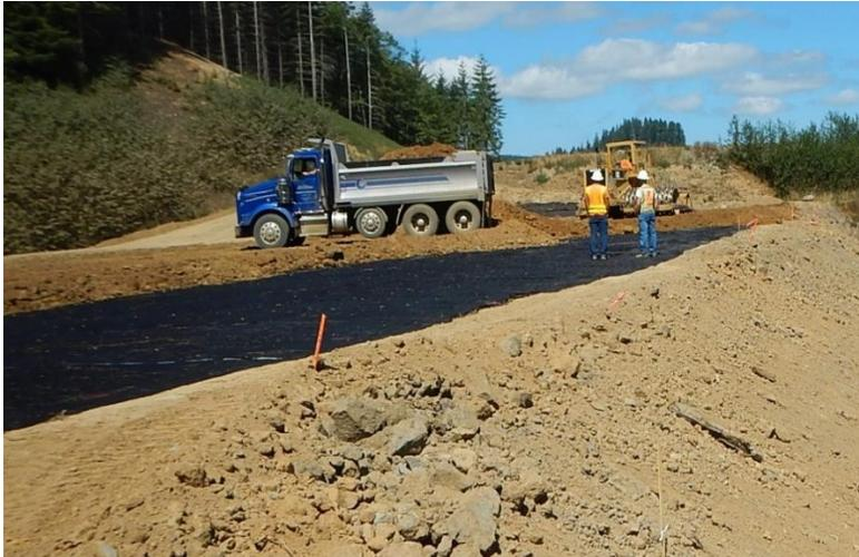
Constructing embankment layered with reinforcing geogrid will prevent the mass landslide known as the deep rotational slump.
