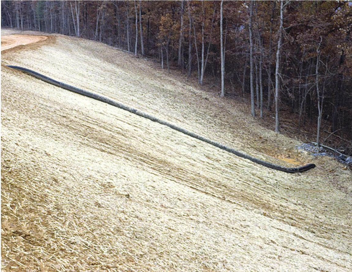
**Figure 3-14 Temporary Slope Drains**
