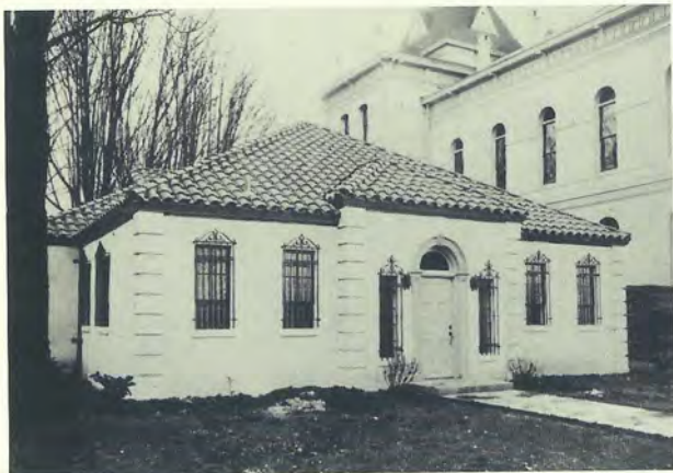
Top: Vault at the west end of the basement. Bottom: The new jail, built in 1929, served until its replacement in 1976.
