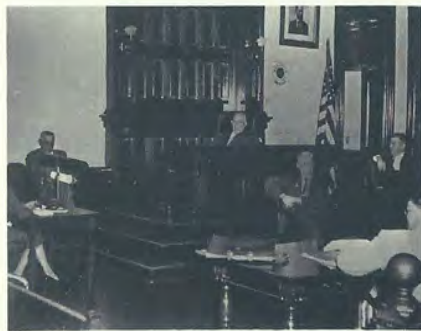
Top: Victor Moses (in the foreground) as County Clerk. Much of the furnishings in this photo have been preserved and are in the Courthouse's new historical display: "The Centennial Room" Bottom: Victor Moses, seated in foreground, in his later years as County Baliff.
