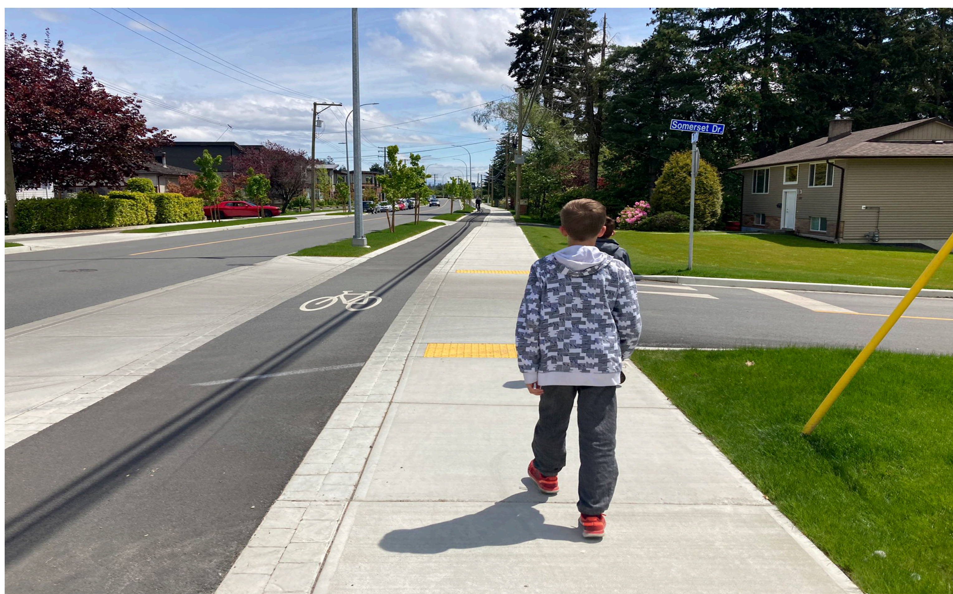
Street View of a Raised Pedestrian and Bicycle Crossing at a Side Street
