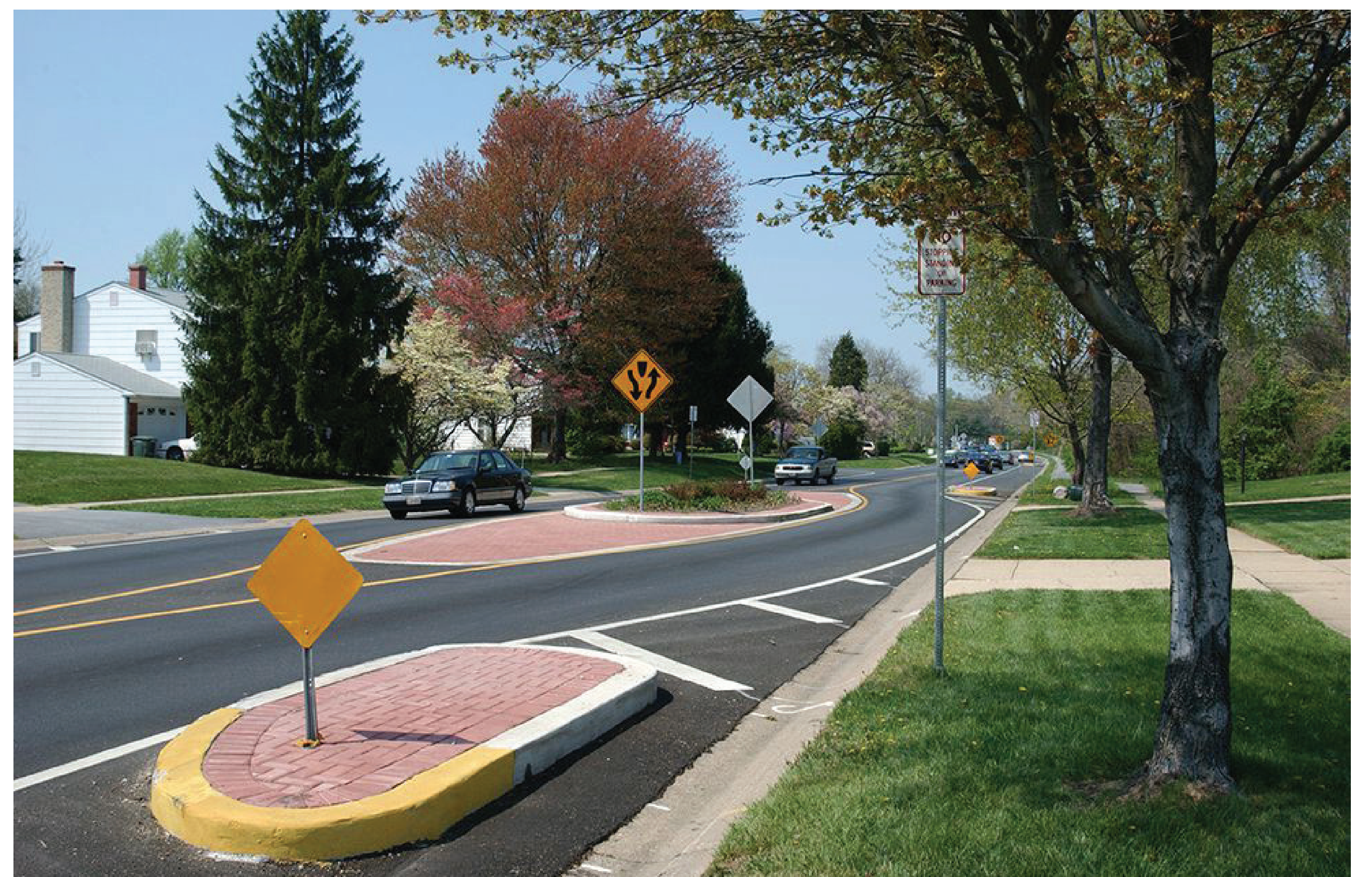
Lane Curvature With Raised Median
