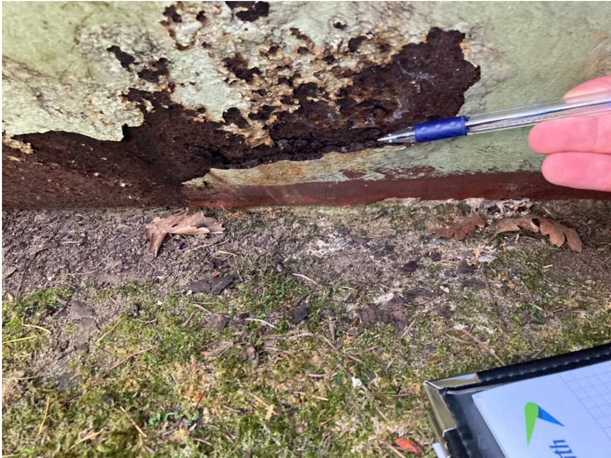
Figure 5-7 Storage Coating Failure
