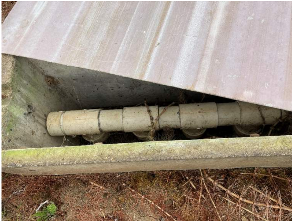
Figure 3-6 Distribution Box with Lid
