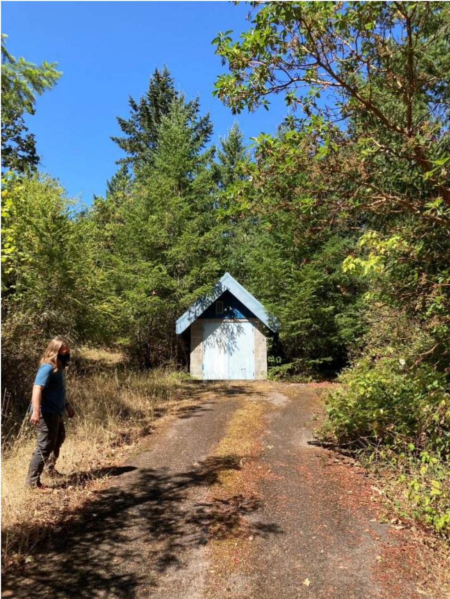
Figure 6-2 Well 1 Well House Exterior
