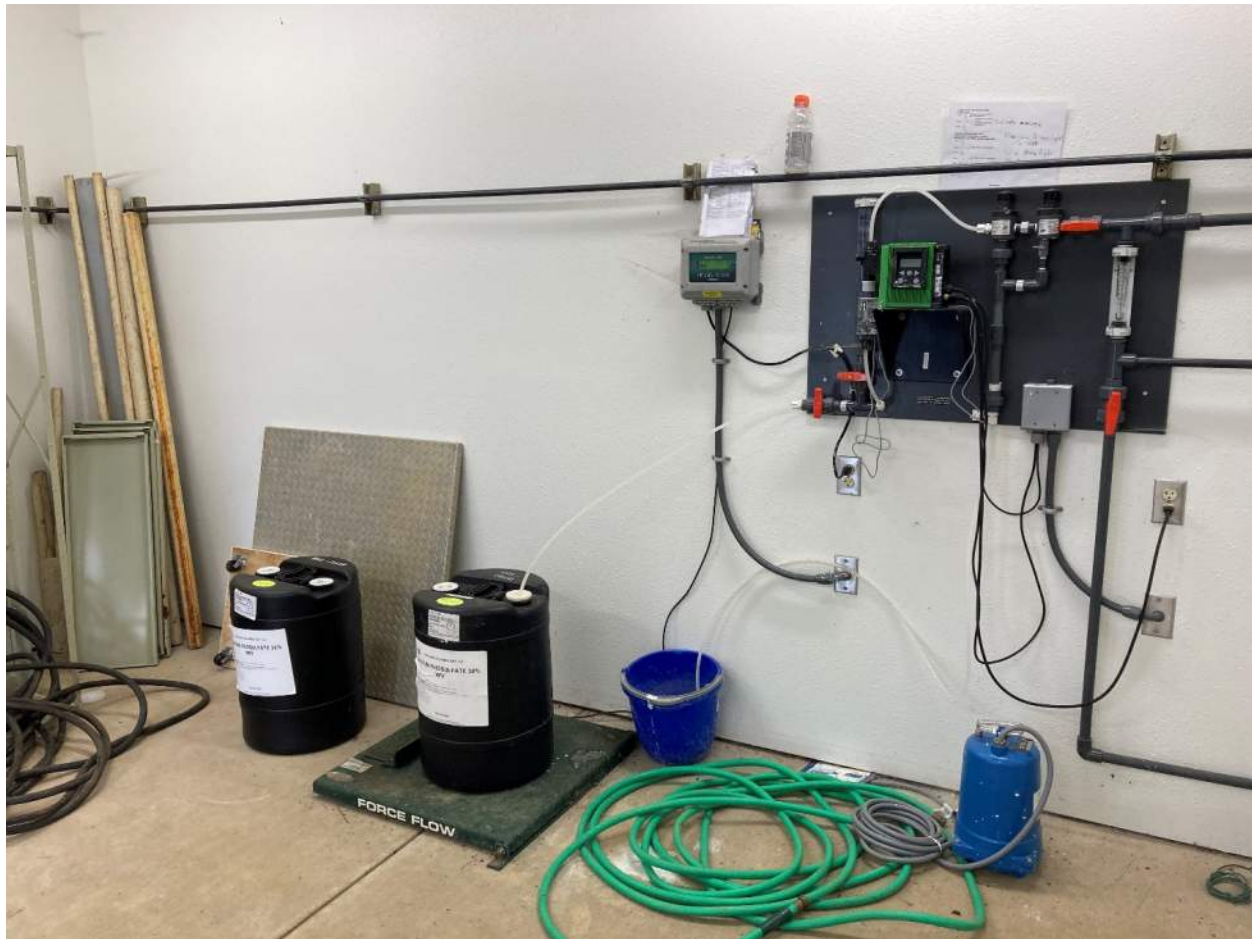
Figure 2-7 Dechlorinate system
