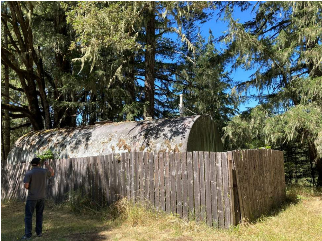
Figure 5-5 Hidden Valley Storage Tank
