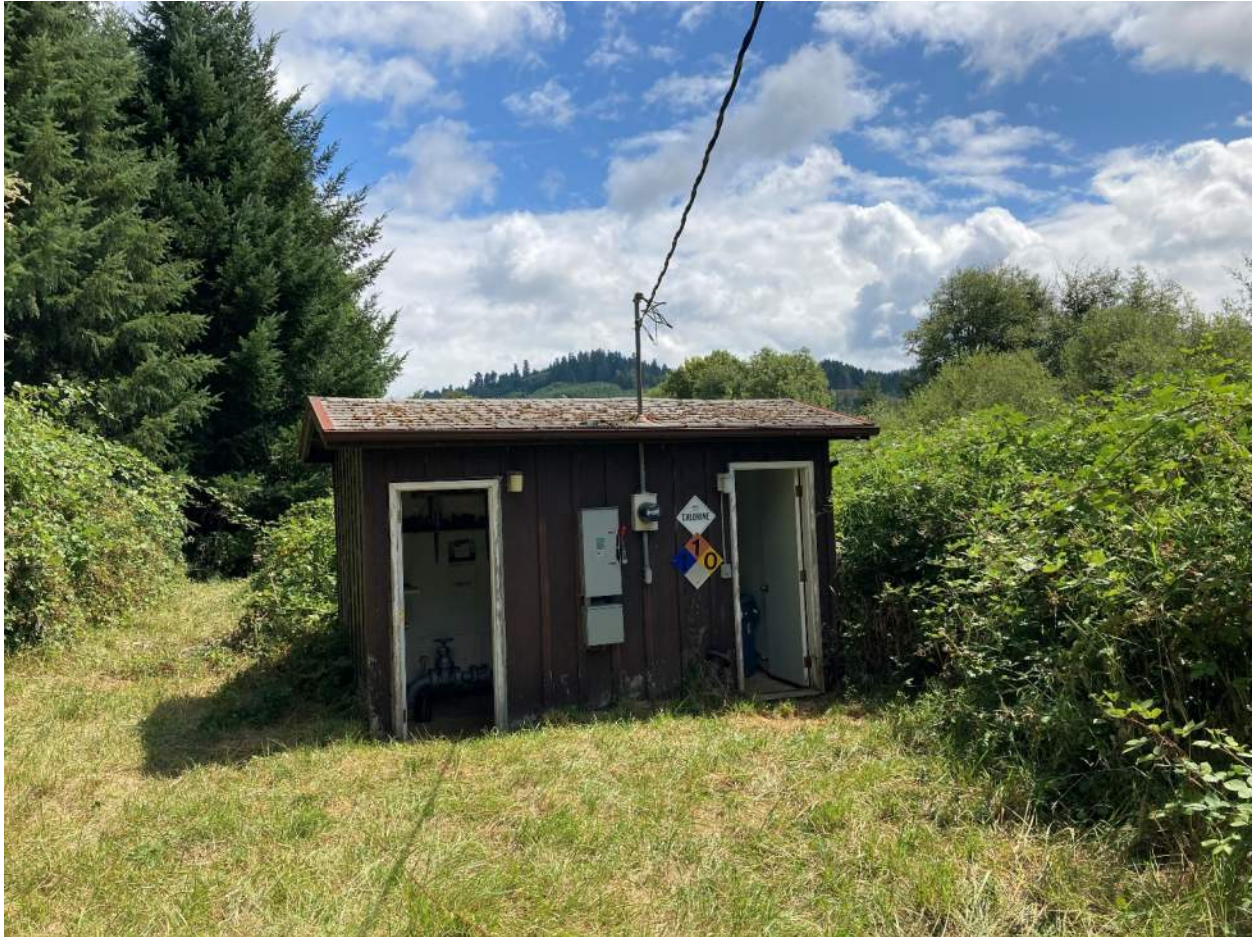
Figure 4-3 Alsea Well House
