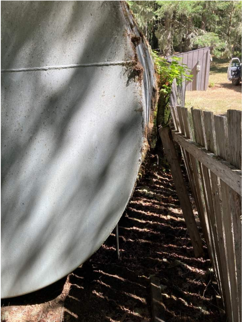
Figure 5-6 Hidden Valley Storage Tank and Fence
