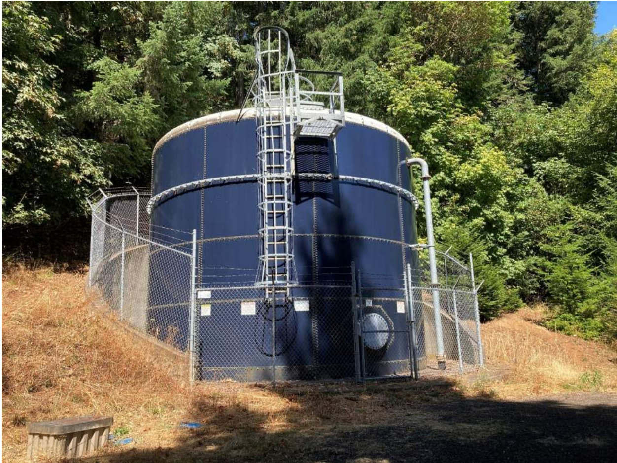
Figure 6-7 Cascade View Storage Tank
